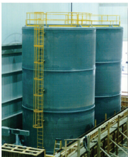
Field Erected FRP Tanks
