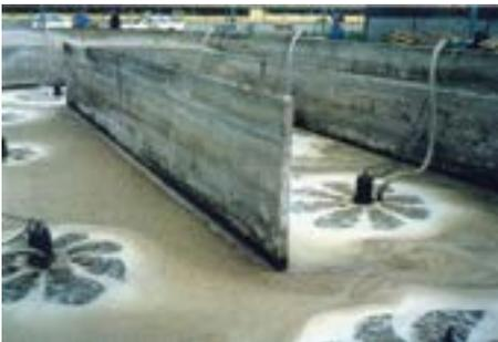
Submersible aspirating aerators ranging in size from 1HP to 55HP. The TRN provides very high oxygen transfer efficiency and mixing.
