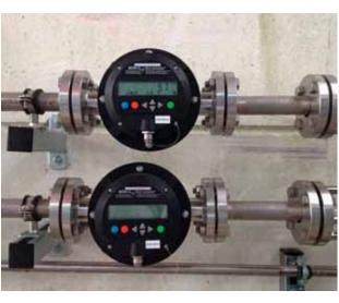
FMO 150 with flange connection installed in a pipeline.
