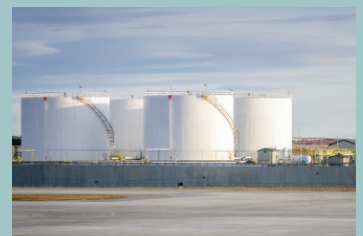
Tank to Tank
