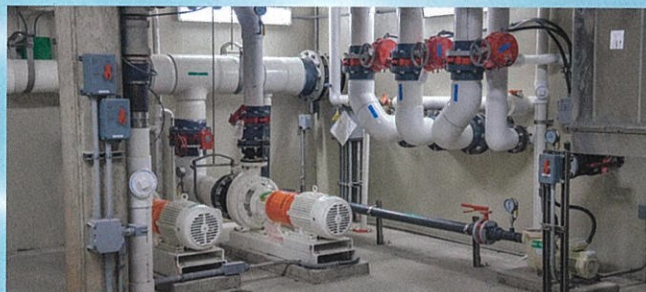
The jet pumps are set on a timer to turn on and scour the bottom of the outdoor exhibit to remove debris.
