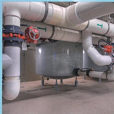
▲ The system includes five sand filters that remove fine solids from the recirculating water.
