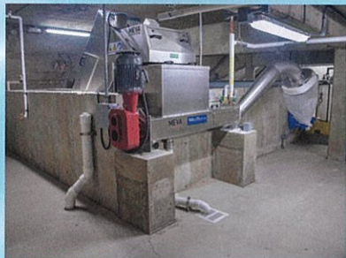
A press squeezes the water out of the waste to allow for the removal of a lighter product.
